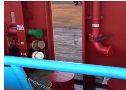
Figure 2: An example of high risk hose connections typically found on board ships
