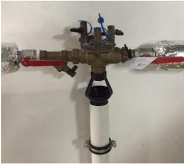
Fig 10: reduced pressure zone (RPZ) valve
