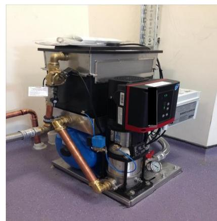
Fig 2: Storage cistern (break tank) supplying school laboratory
