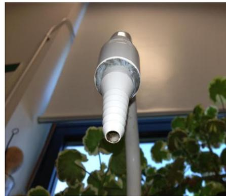
Fig 9: Any obstruction or interference with the air apertures, such as taping up or plugging, will eliminate the backflow protection placing the water supply at risk
