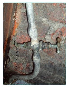
Figure 5 – Example lead pipe arrangement
